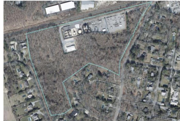
A battery energy storage system caught fire in May at the electrical substation
